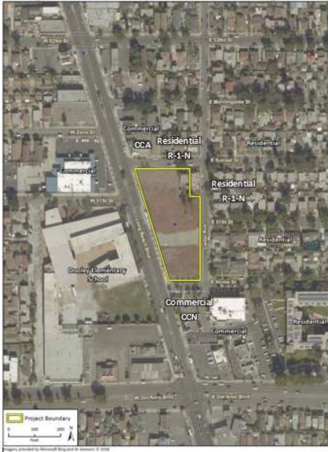
Figure 1: Aerial of Project Site and Surrounding Uses
