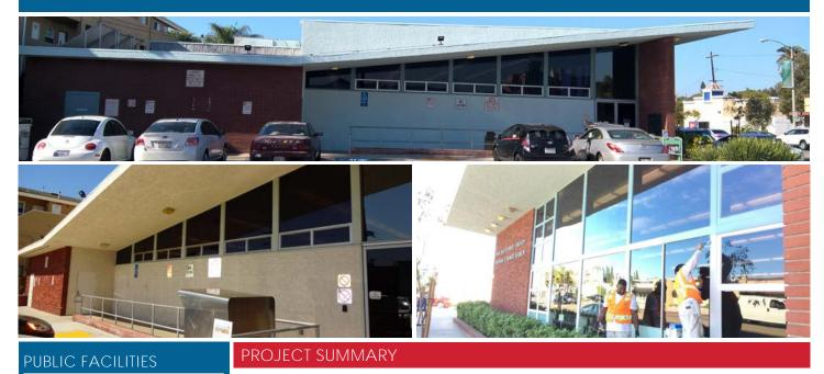
The Brewitt Branch Library project removes and repairs flaking paint around windows, and paints exterior features.
