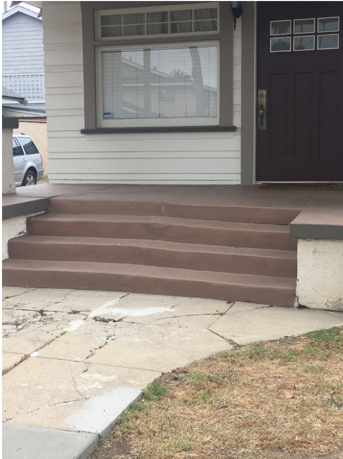
Front Porch - foundation failing
