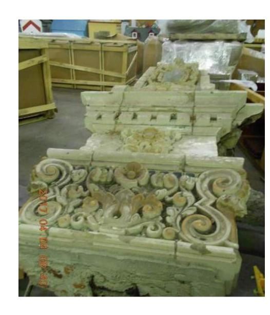
**Figure 12.** Typical terra cotta piece from parapet. Source: Jergins Trust Artifact Inventory, 4/4/17, courtesy of GBD Architects.
