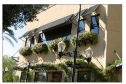
Solar orientation of the building, overhangs, and other devices placed on the exterior of buildings reduce direct sunlight into interiors, lowering heat gain and the amount of energy needed for cooling.
