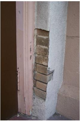
Original Brick Beneath Stucco on West Elevation
