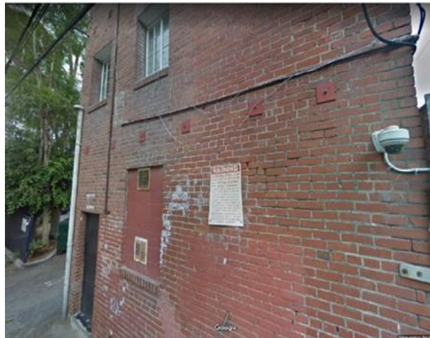
Photograph 5: Close up of the ground floor of the west elevation (rear). Note the replacement rick work and bricked up original window opening. View north (Google Earth 2023).
