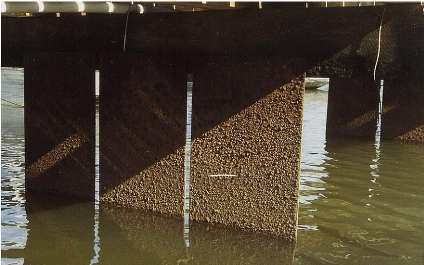
**Fig. 2.** Corroded surfaces of steel plates under jetty after 6 months splash and tidal zone exposure showing uniform nature of external rust layer. [SCAN0042a.jpg.
