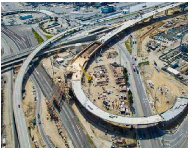
Freeway interchange in Long Beach
