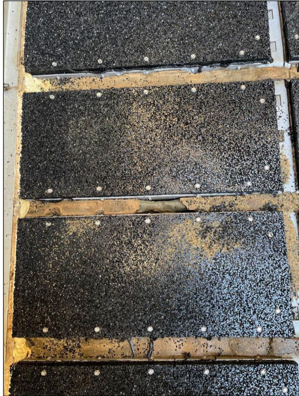
Missing grout between porous caps
