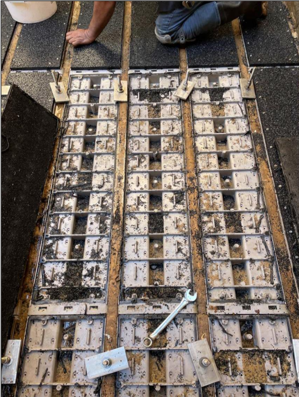
Gasket material and media found under porous cap
