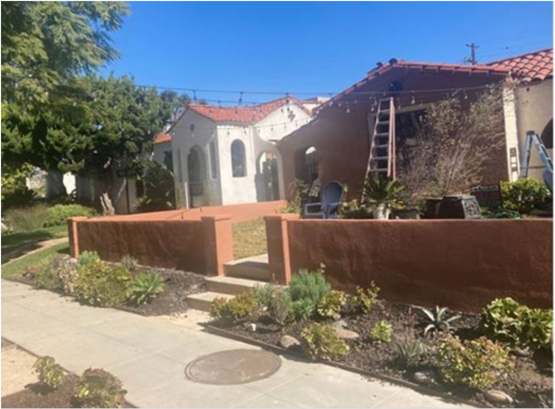
February 23, 2022 – Paint is completed.
