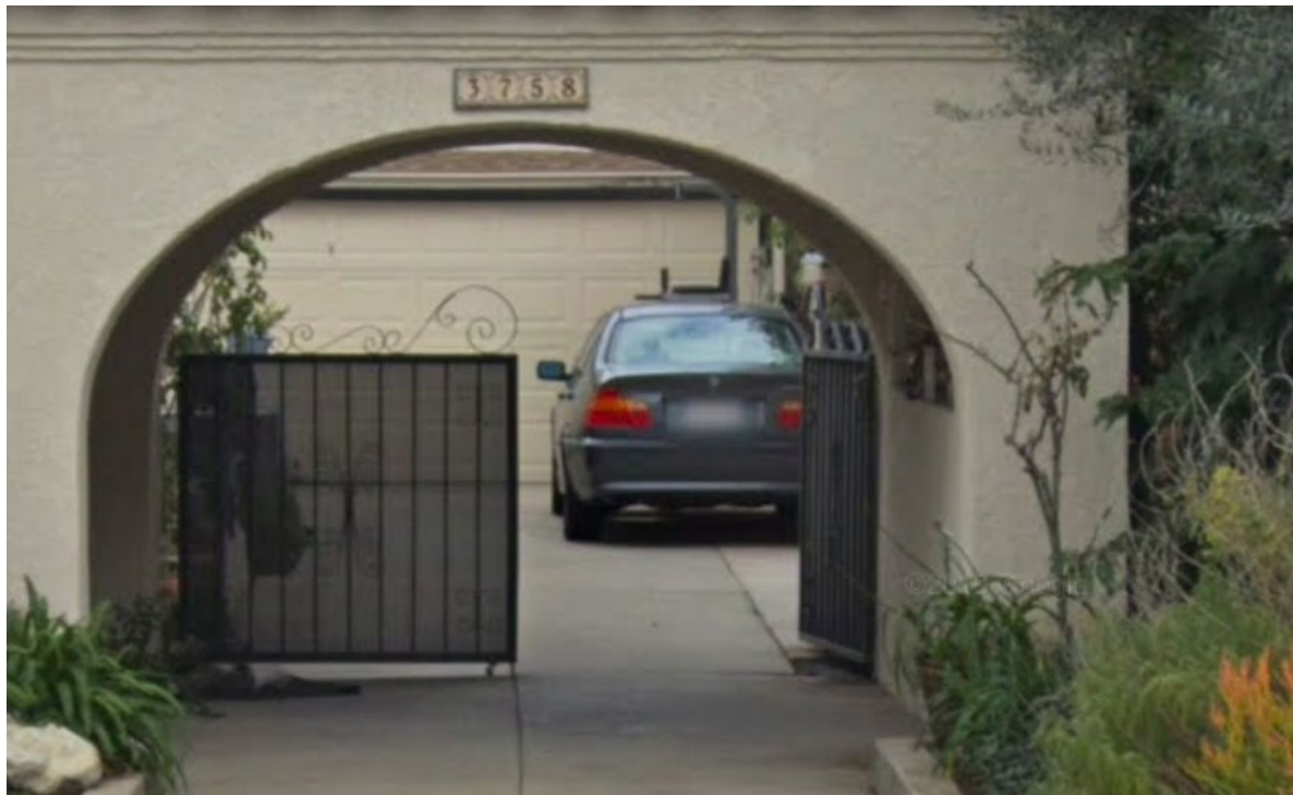
Driveway gate installed at rear of porte-cochère.
