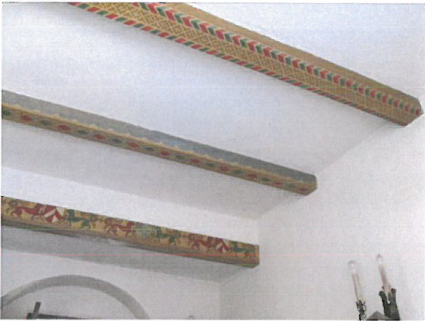
Image 19: Second floor hall ceiling detail
