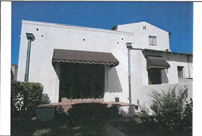
Image 9: South elevation, looking northeast
