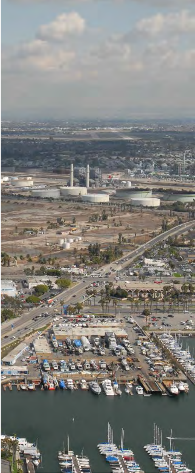
Wetlands in the SEASP are located in close proximity to existing roadways. As such, changes to roadways are primarily limited to changes in lane and striping configurations within the existing right of way.
