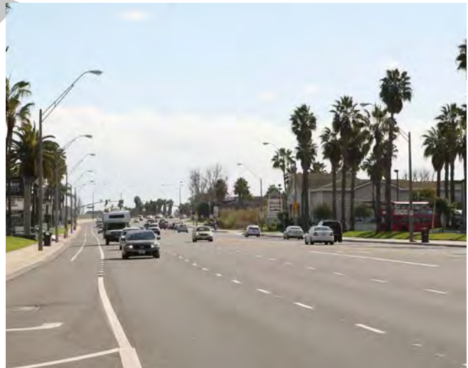
Much of the supporting infrastructure for the SEASP area runs under major thoroughfares such as 2nd Street, Pacific Coast Highway, and 7th Street.
