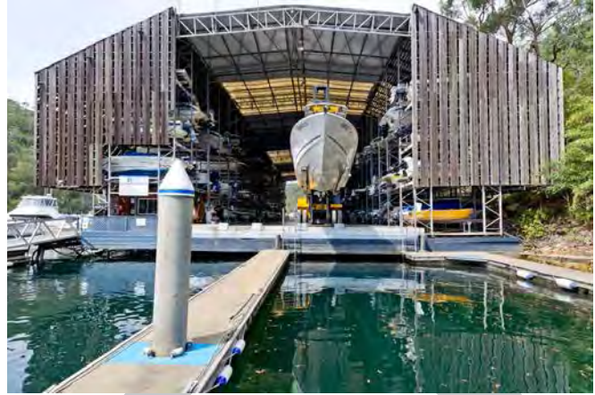
Well designed boat storage facilities should screen views of service areas. Photo Credit: d'Albora Marimas
