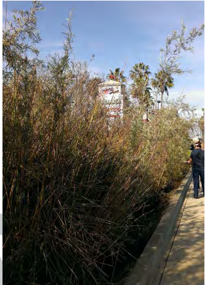
Low impact development measures such as this bioswale at the perimeter of the Marina Shores Shopping Center, are a best management practice for runoff capture, and biofiltration in the SEASP area.
