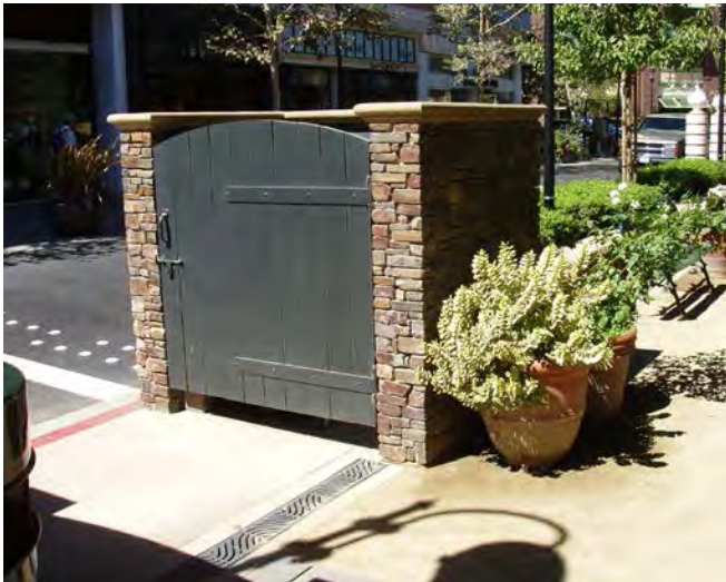
Brick and wood screen for utility area.
