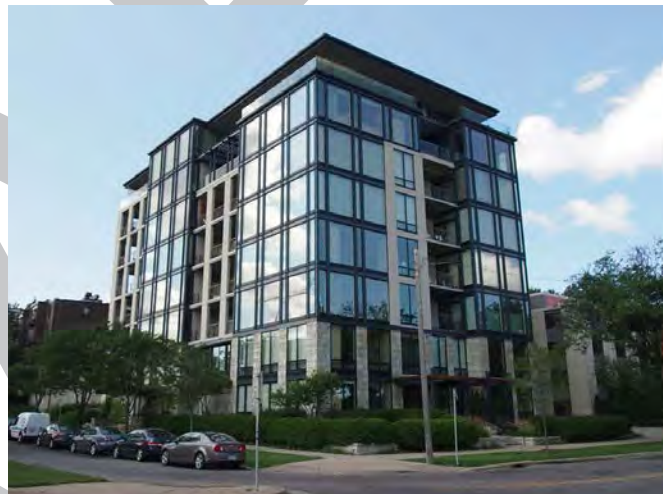
A 7-story high-end building uses modern materials and details in a sophisticated manner to appear as light as possible and to capitalize on views to a popular park and major museum across the way.
