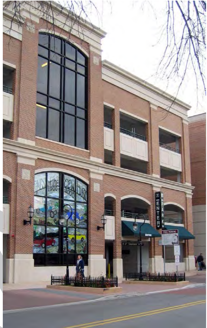
Entrance to a parking structure.
