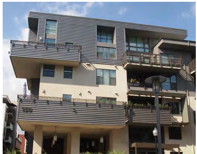
Balconies that shield visibility of personal items from public view.
