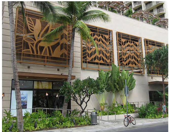
Parking structure screened with decorative panels.
