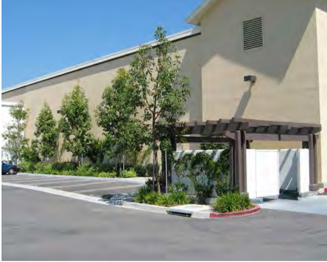
Pergola used to screen utility area.
