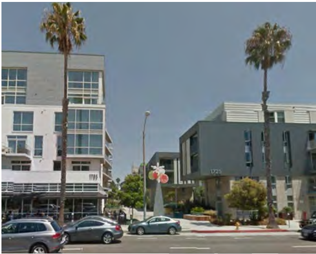
The buildings feature variation in massing and facades while framing a large paseo with public art. These buildings reflect an emphasis of human scale elements and accessibility. Source: Google Earth Pro
