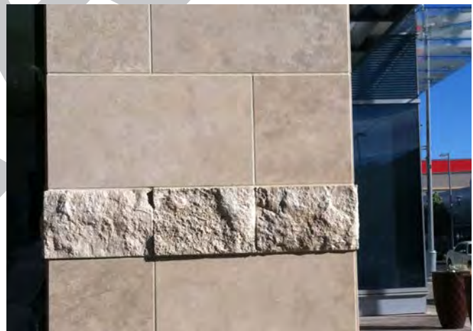
Materials shall vary in the vertical plane. Buildings shall exhibit greater detail and higher quality materials at the lower levels, where viewed by pedestrians.
