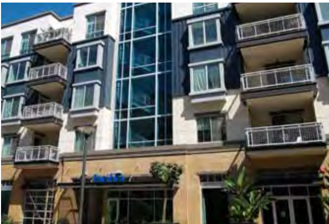
Windows and doors are a part of a comprehensive approach to massing and elevation design. Shown above are inset details, bay windows, taller ground-floor storefronts and emphasis on the pedestrian lobby entrance.
