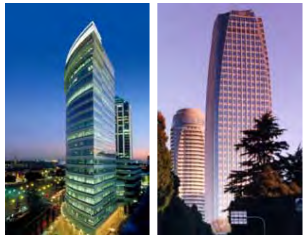
Example of office towers with high-quality materials, simple forms and a distinct manner of how they taper or meet the sky. Note that even transparent or clear glass will reflect some sky; the more reflective mirrored coatings are not encouraged.
