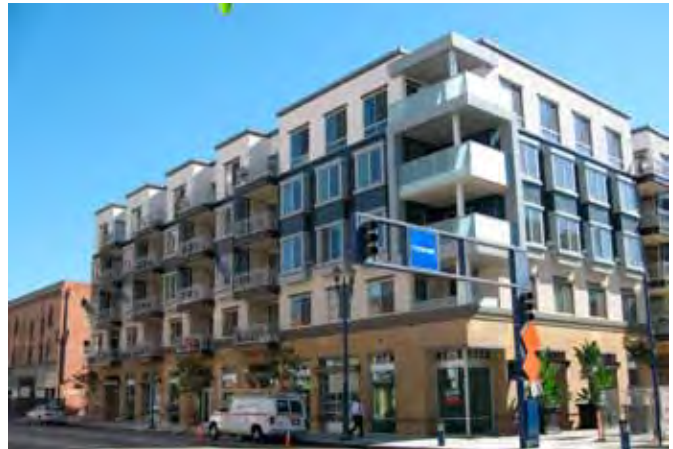
Example of low-rise mixed-use project with massing and materials that delineate balconies, building corner and ground floor.
