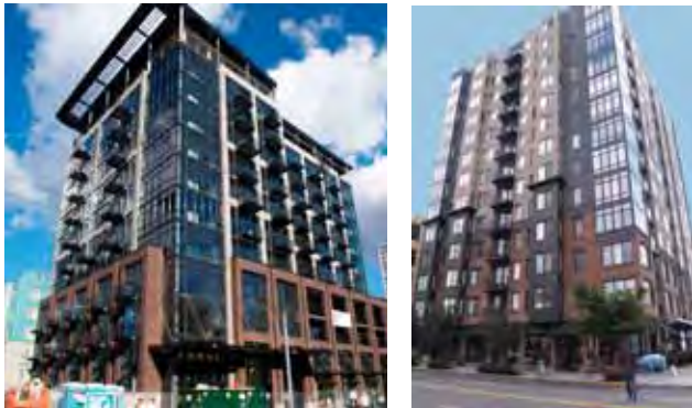
Brick focused at lower levels, transparent upper floors, metal detailed balconies and penthouse sun shading element create an innovative industrial style for this mixed-use building. At right, a traditional brick exterior is used at the lower levels in combination with metal panels and concrete to achieve a modern aesthetic.
