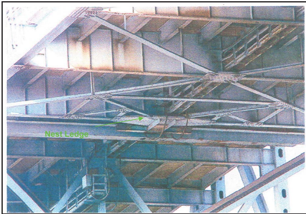
Exhibit 2.3.5-1 Peregrine Falcon Nesting Ledge on the Existing Gerald Desmond Bridge
