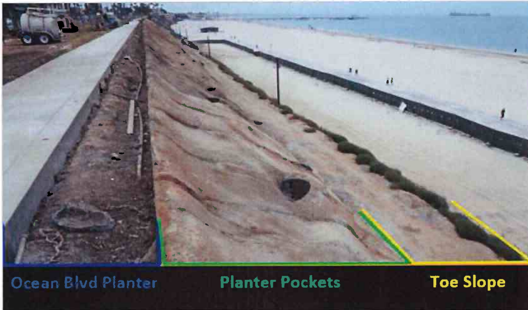
Figure 5. Planter Delineations before plant installation
