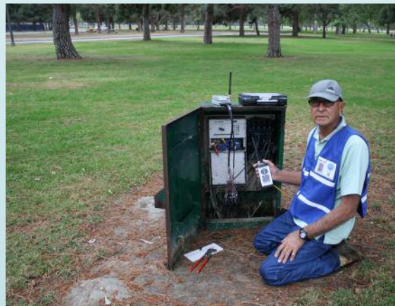
Certified Landscape Water Auditor (CLIA), John Oudyk sets up controller for remote operation
