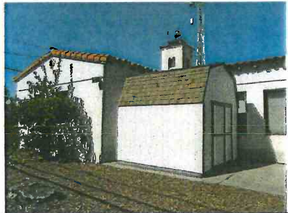
Photo 7: South elevation, west end, view northwest.
