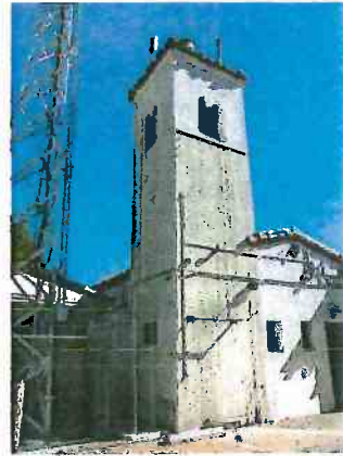
Photo 5: Detail of tower, view southeast.
