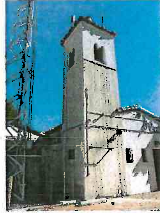
Photo 5: Detail of tower, view southeast
