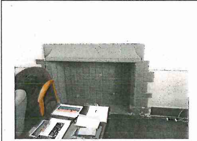
Photo 8: Fireplace detail, view south.
