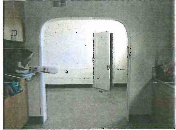
Photo 9: Arched doorway in kitchen and dining room, view west
