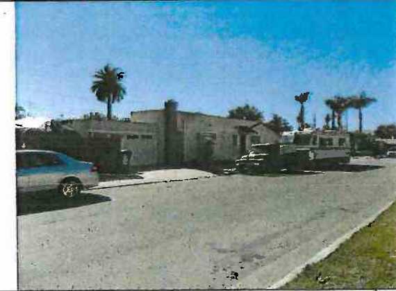
Photo 19: Properties southwest of Fire Station No. 12 on 65 th Street, view southwest
