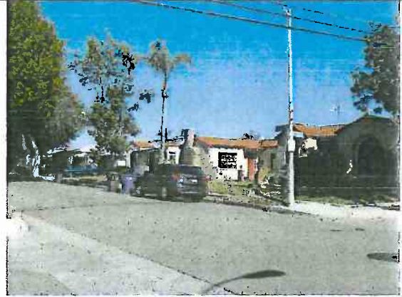
Photo 15: Properties directly east of the Fire Station on Gundry Avenue, view northeast.
