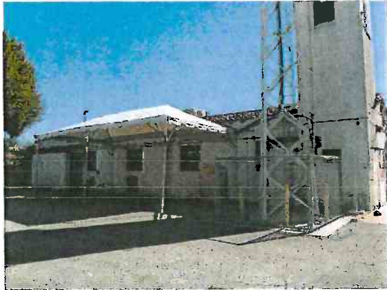
Photo 4: North elevation, view southeast
