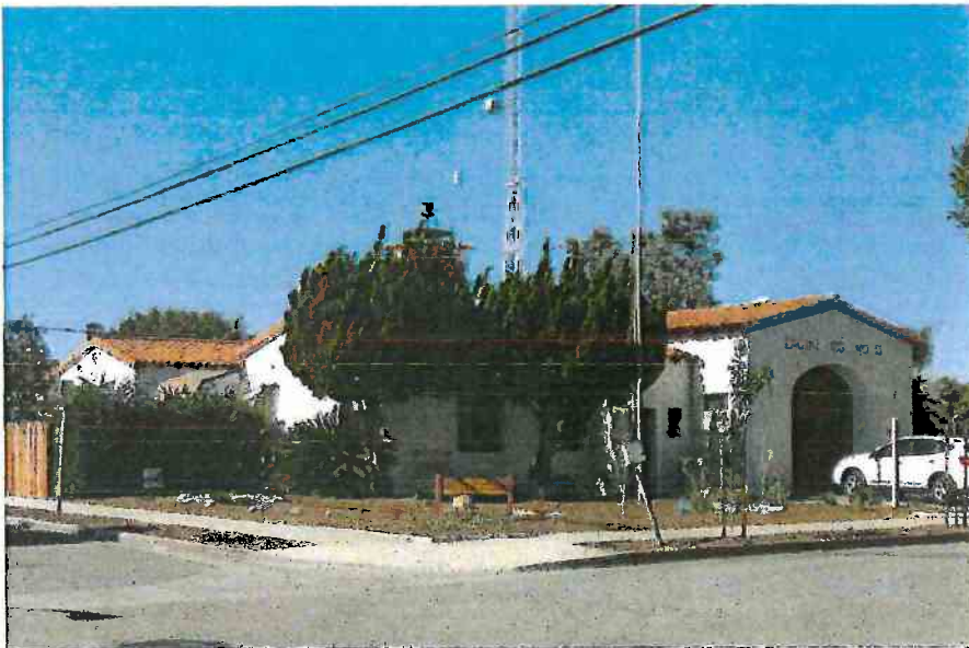
Photo 1: East facing façade (right) and south elevation (left), view northwest
