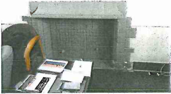
Photo 8: Fireplace detail, view south
