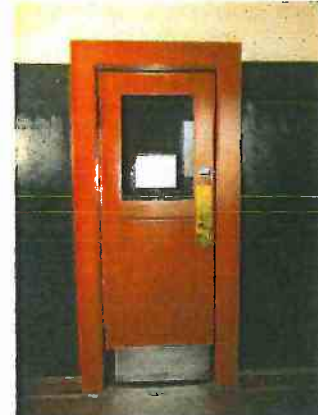
Photo 13: Interior door leading to locker room
