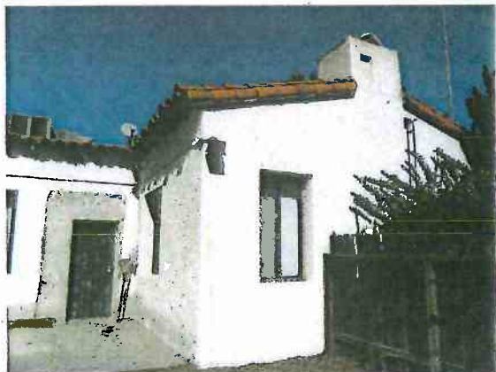
Photo 6: South elevation, east end, view northeast.
