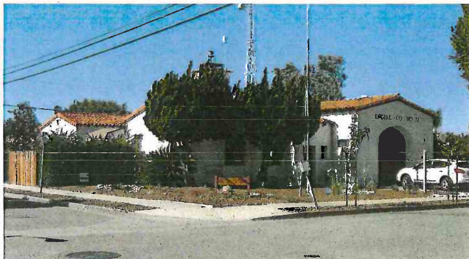
Photo 1: East-facing façade (right) and south elevation (left), view northwest.
