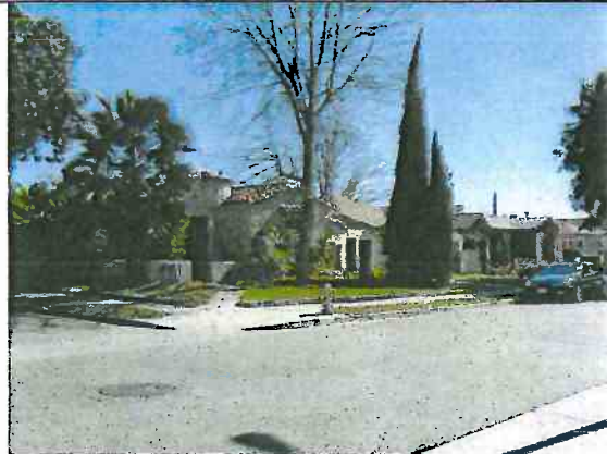
Photo 16: Properties southeast of the Fire Station on Gundry Avenue, view southeast.
