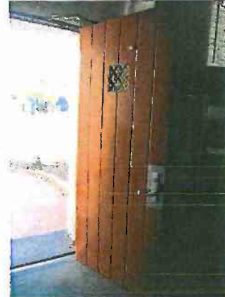
Photo 11: Front door detail
