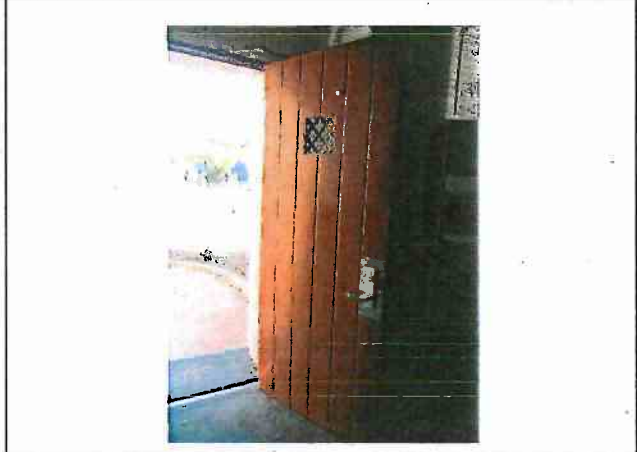
Photo 11: Front door detail.
