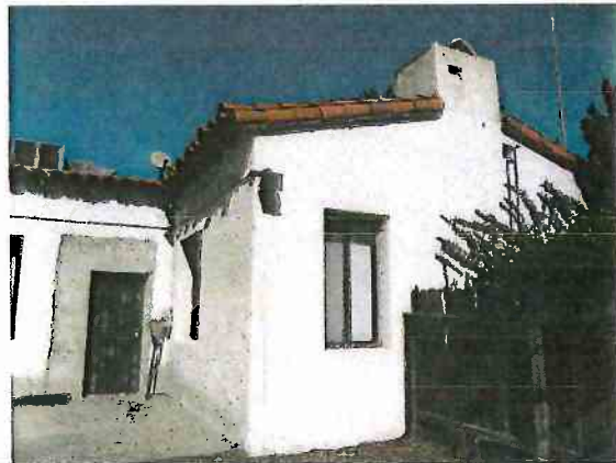
Photo 6: South elevation, east end, view northeast
