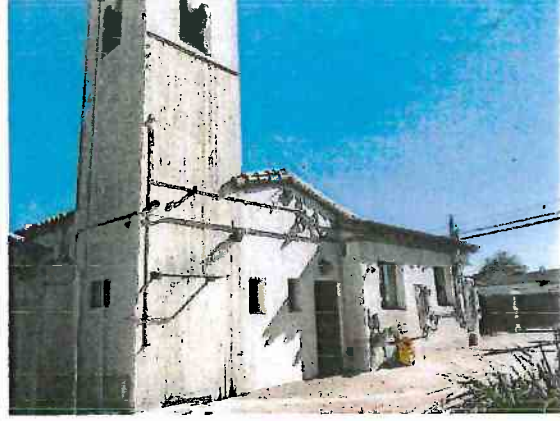
Photo 3: West elevation, view southeast
