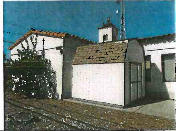
Photo 7: South elevation, west end, view northwest
