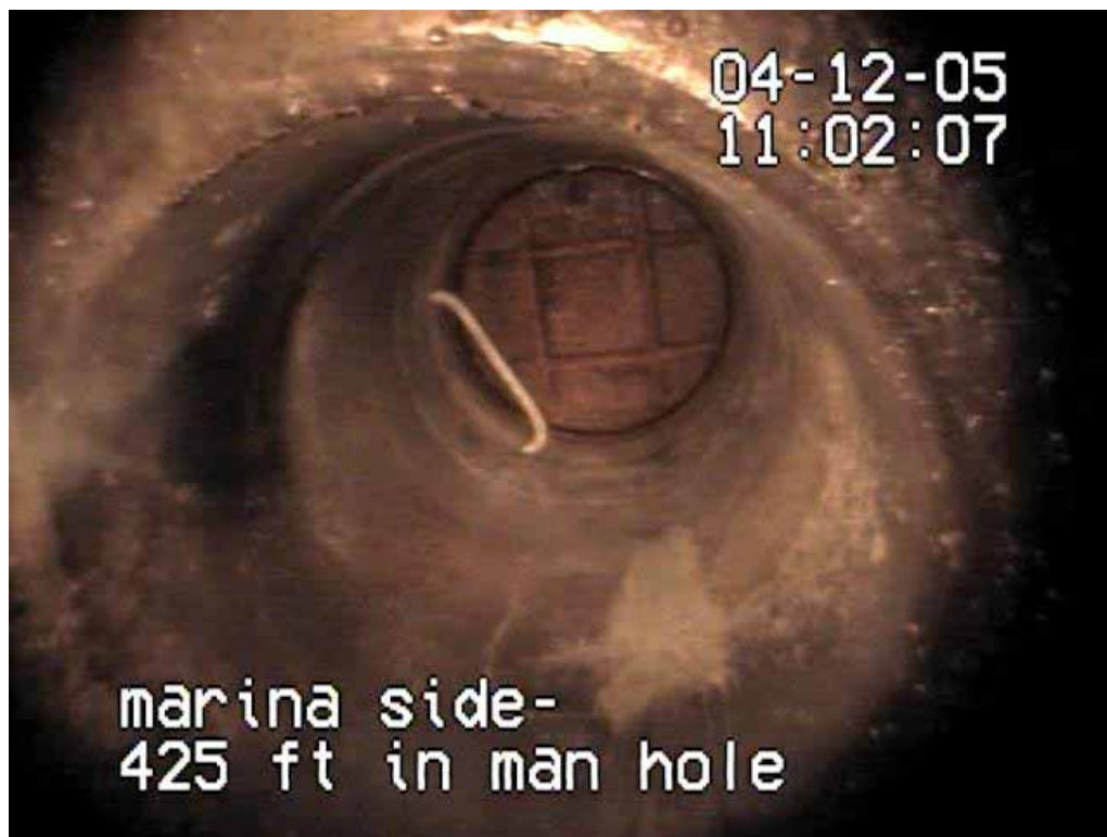
PHOTO 4 - VERTICAL SHAFT AND MANHOLE ACCESS AT 425 FT IN FROM MARINA SIDE
