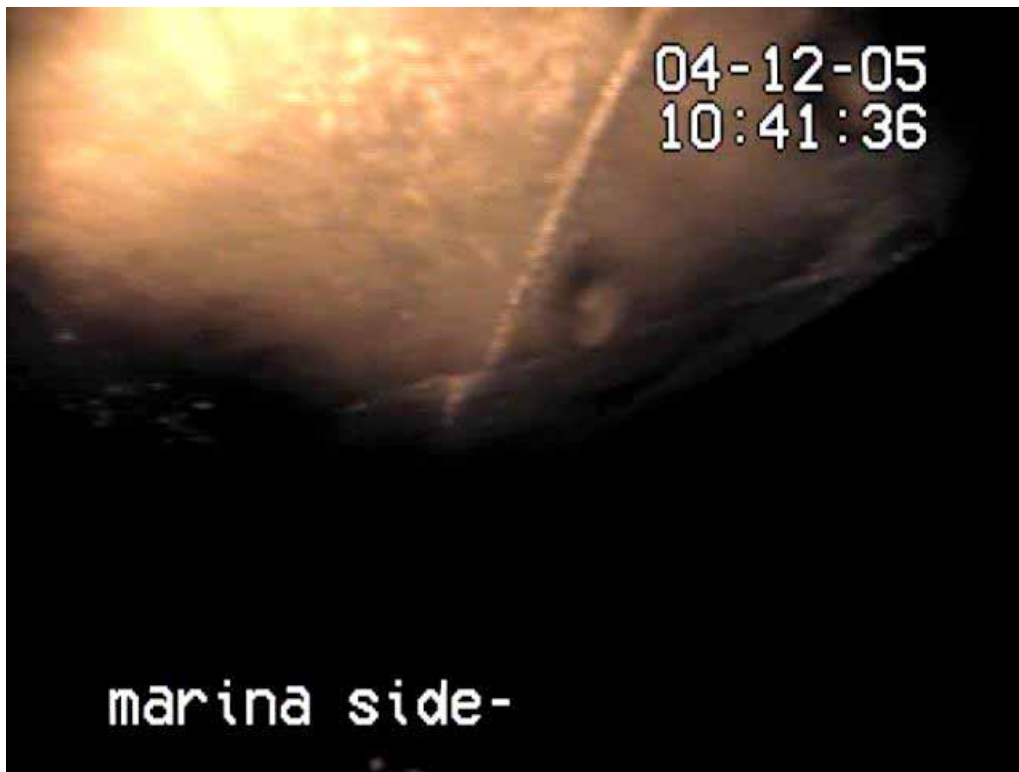
PHOTO 1 - TYPICAL CLEAN TOP OF CULVERT WITH NO BIOFOULING
