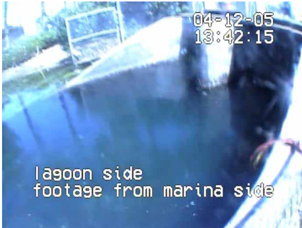
PHOTO 7 - LAGOON OUTLET STRUCTURE SHOWING THE WING WALL AND DIVIDER WALL
