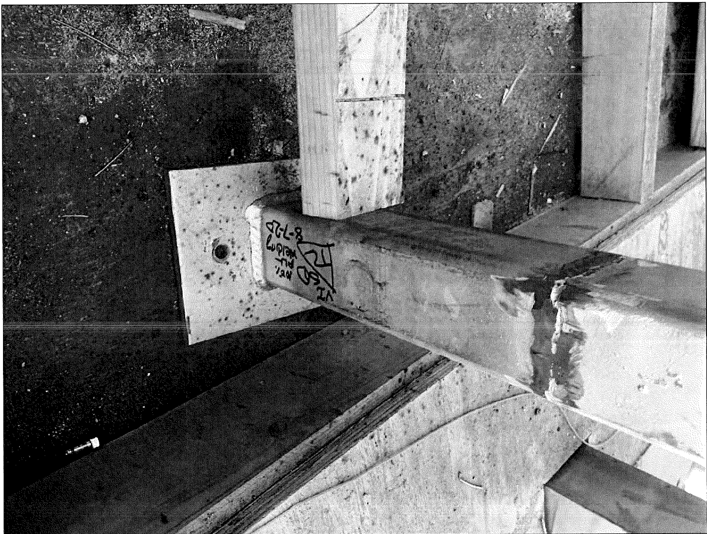
Completed weld and Inspector markings
