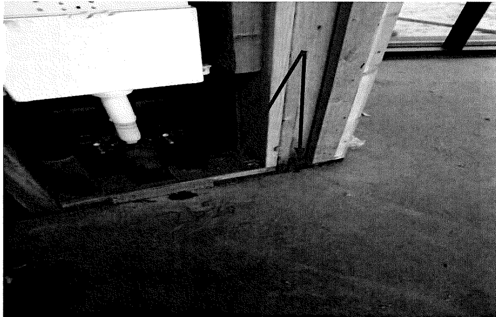
Anchor bolt missing
