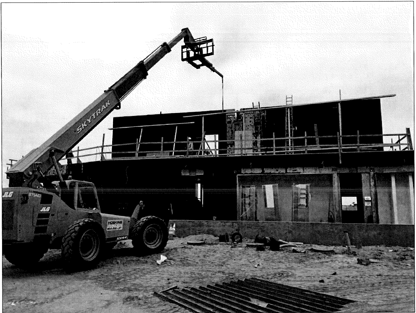
Erecting Mechanical Screen Framing
