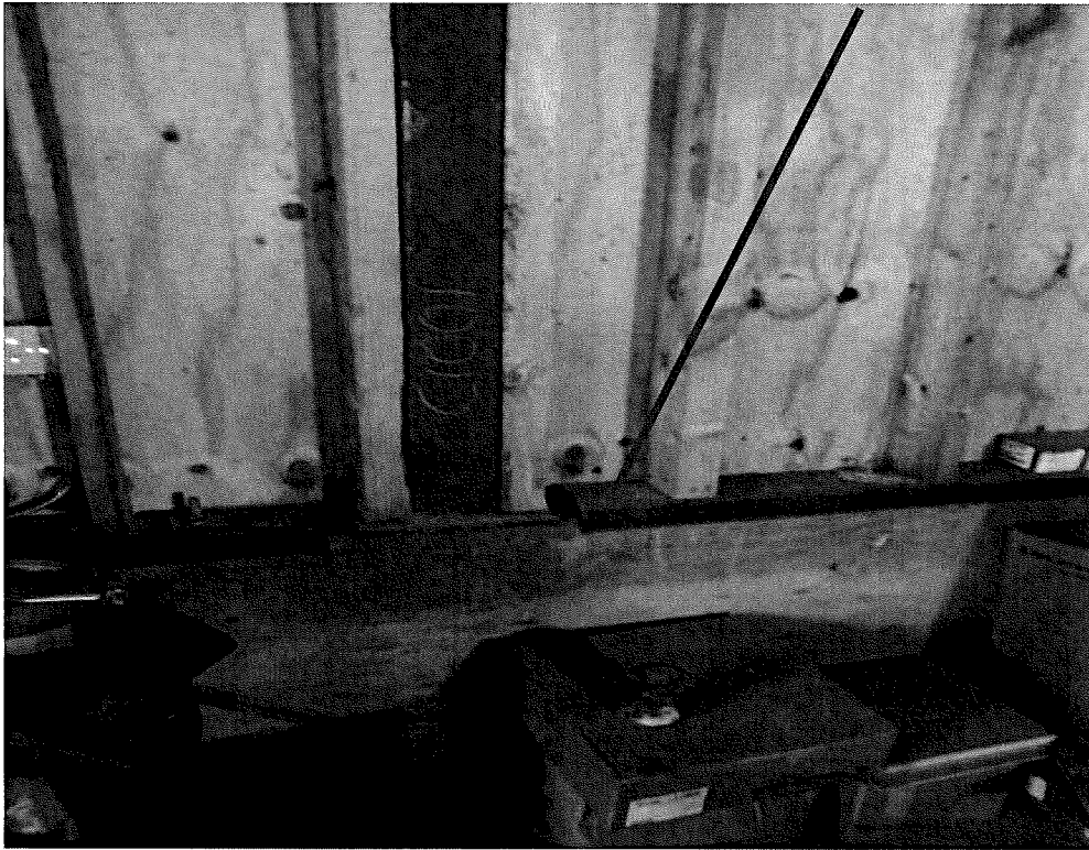
Anchor bolt missing
