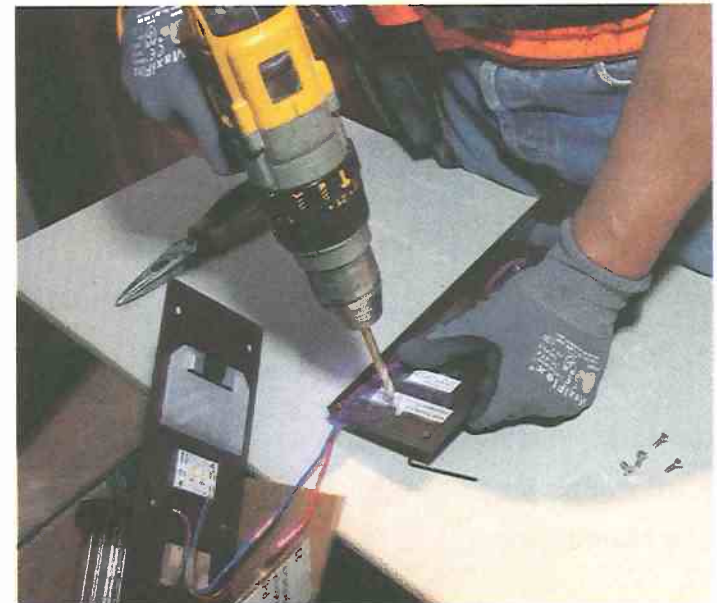
Installing a hallway light fixture.
