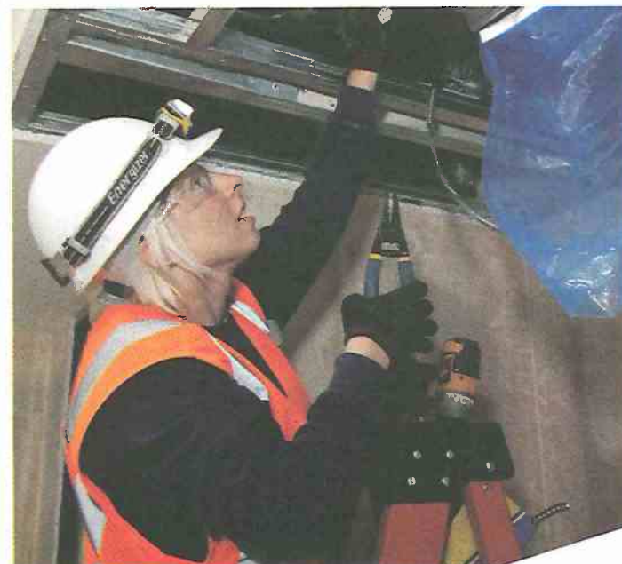
Installing a hallway light fixture.
