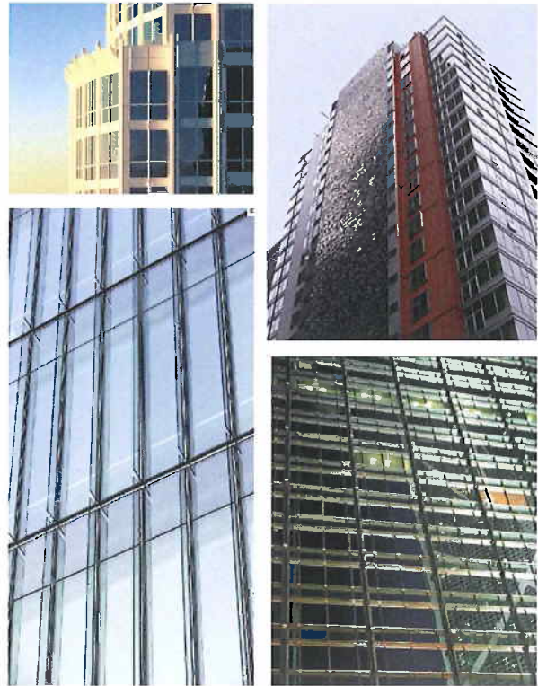
Example of constructed towers (clockwise from upper left): Commercial tower with sophisticated curtain wall, divided windows and vertical fins; coated metal panels introduce color into this residential tower; two curtain wall systems that add another layer of texture with a metal frame, and glass fins.
