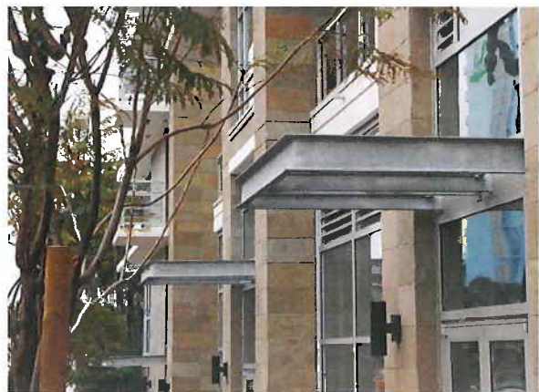
Example of a setback elevation that uses some variation in heights, balconies and materials; the windows and doors are well detailed and noticeably inset. Example of higher quality materials and entrance canopies being used at the ground floor.
