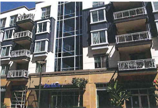
Windows and doors are a part of a comprehensive approach to massing and elevation design. Shown above are inset details, bay windows, taller ground-floor storefronts and emphasis on the pedestrian lobby entrance.
