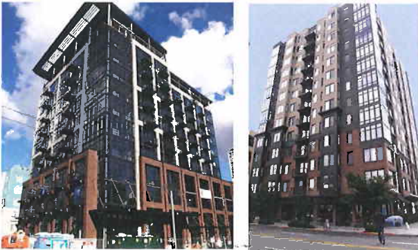
Brick focused at lower levels, transparent upper floors, metal detailed balconies and penthouse sun shading element create an innovative industrial style for this mixed-use building. At right, a traditional brick exterior is used at the lower levels in combination with metal panels and concrete to achieve a modern aesthetic.
