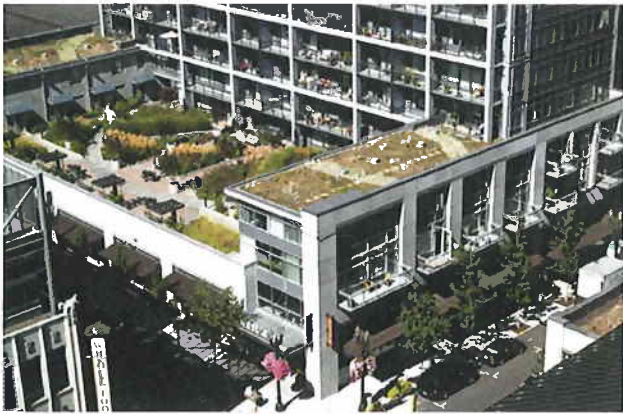
Example of a green roof on the lower floors of a mid-rise building that collects rainwater and provides open space with visual benefits.
