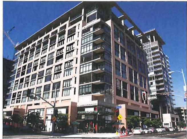
Example of mid-rise mixed-use project that is relatively transparent and interprets the classic building base, middle, and top in a modern way.
