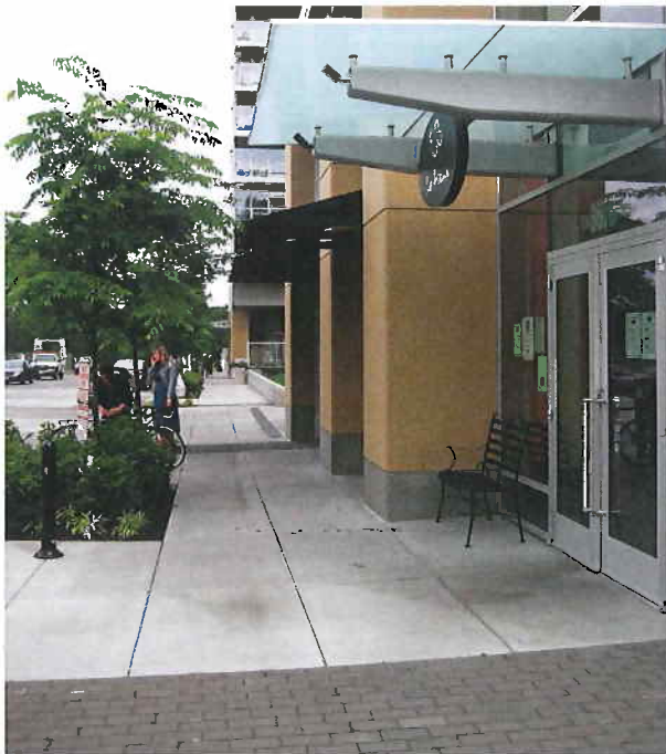
Standard grey concrete sidewalks may be complemented by pavers of a similar color (above) or sawcut in a diagonal pattern (right) to add visual interest.
