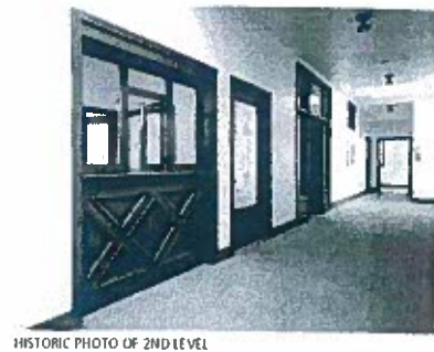
HISTORIC PHOTO OF 2ND LEVEL
