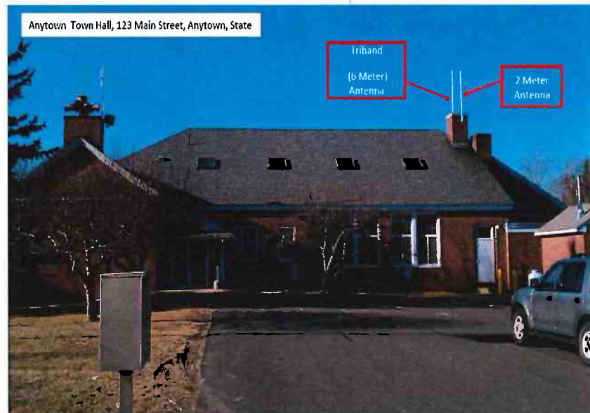
Figure 2. Example of ground-level photograph showing proposed attachment of new equipment
