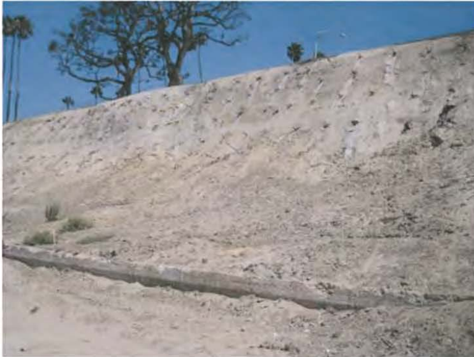
Figure 1 – Existing Slope Condition in Area 1
