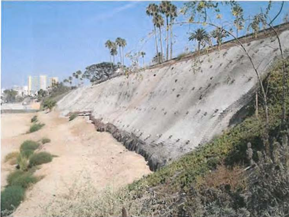
Figure 2 – Initial Layer of Shotcrete in Central/Eastern Portion of Area 2
