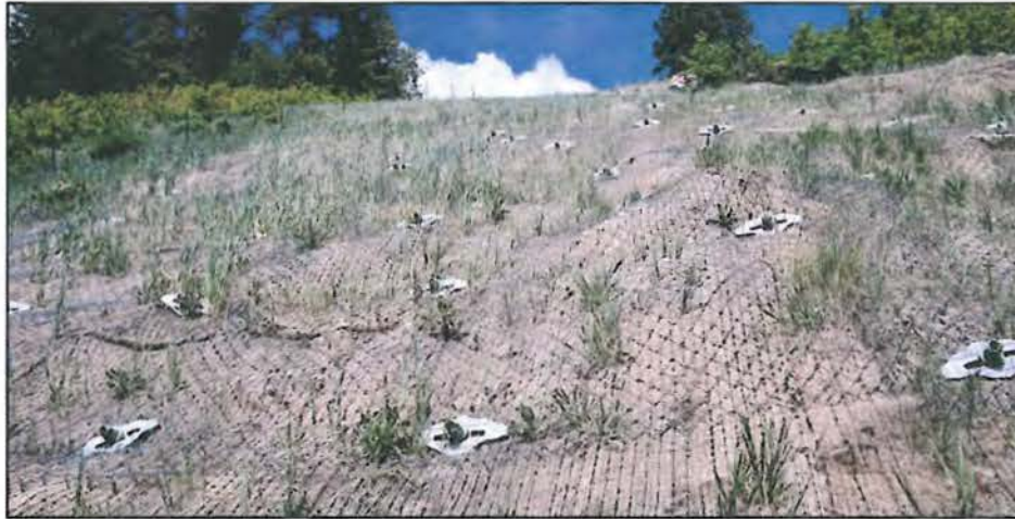
Figure 2. Photo of vegetation growing through Tecco mesh. Source: geostablization.com
