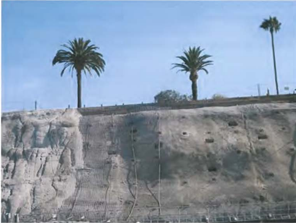
Figure 3 – Transition Zone - Full and Initial Layer of Shotcrete in Area 2
