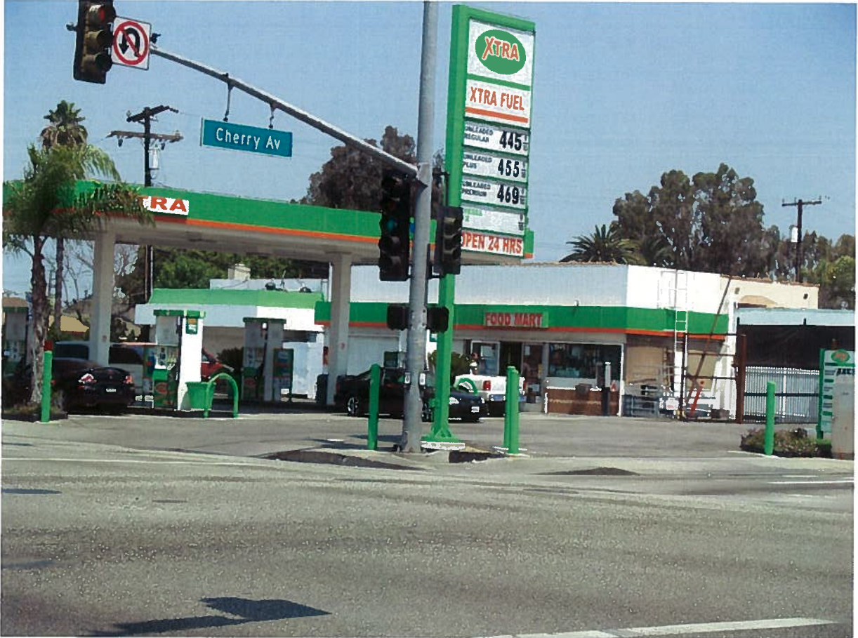
1925 East Pacific Coast Highway (Northwesterly View)
