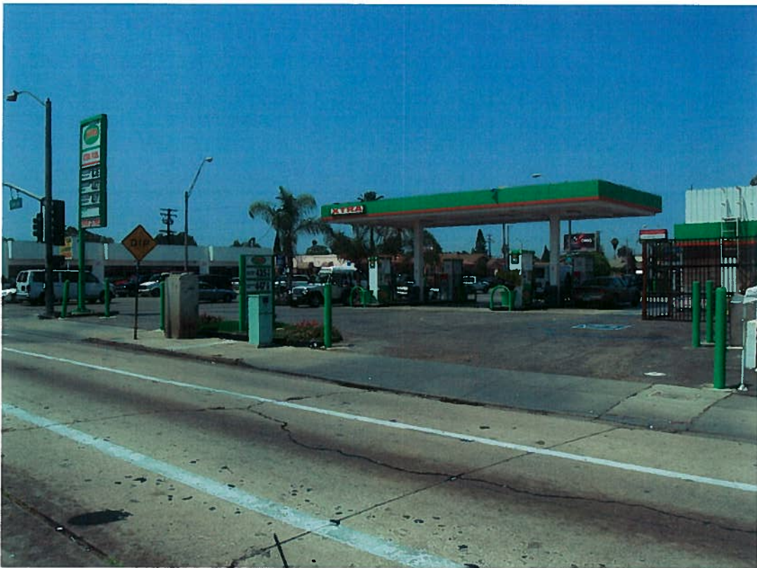
1925 East Pacific Coast Highway (Southwesterly View)
