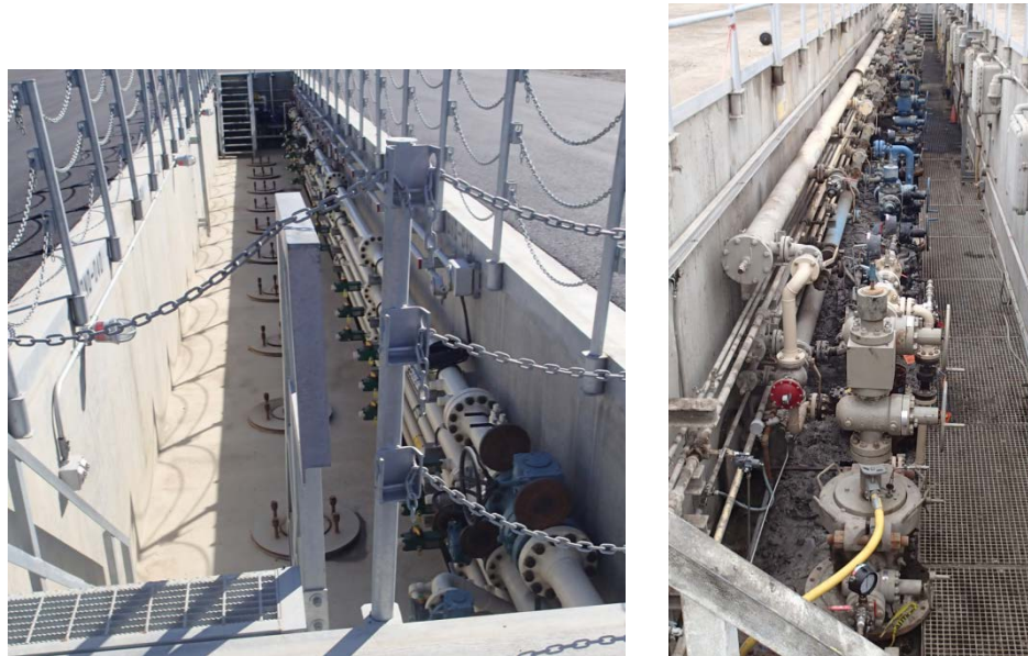
Figure 2: Typical Common Well Cellars
