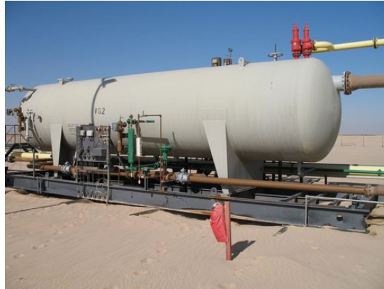
Figure 7: Typical Free Water Knock Out (FWKO)
