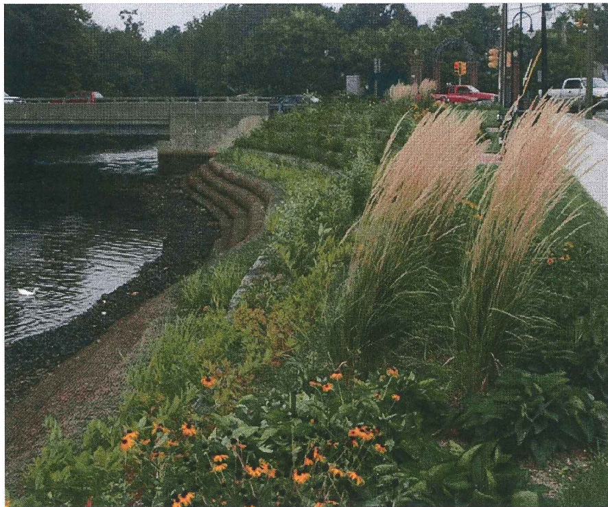
Figure 2 shows an example of a Vegetated Reinforced Soil Slope with a mix
