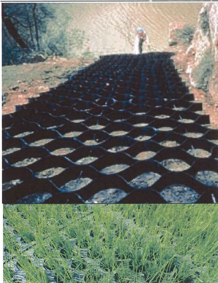
Figure 3. Shows an example of a Geoweb slope protection that allows for vegetation plantings providing slope stability and in an aesthetically pleasing manner.
