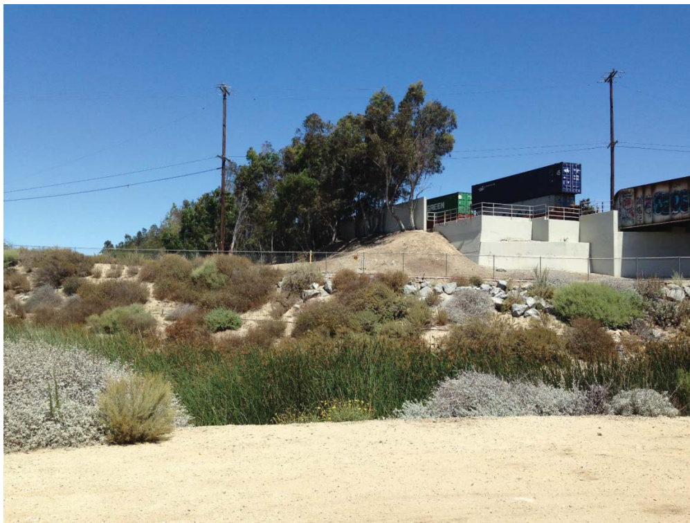
Photo 2: Union Pacific (UP) railroad tracks and train passing along the southern boundary of the project site, with Dominguez Gap Wetlands in foreground.
