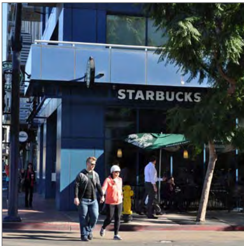
Mixed-use buildings with ground floor retail uses create an active, pedestrian-friendly environment.
