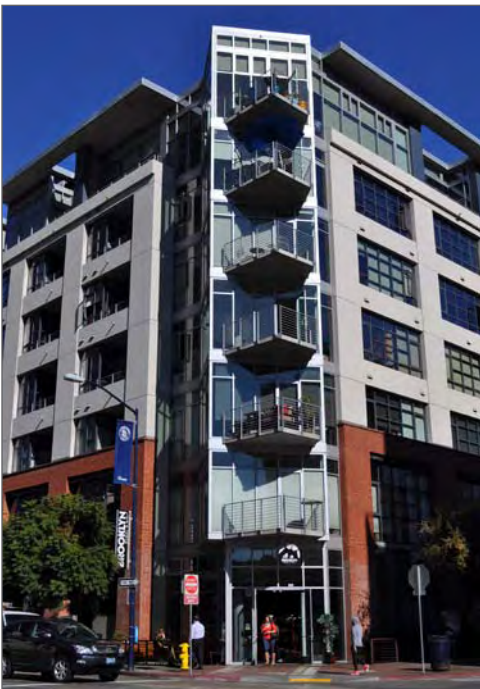
Balconies may enhance a building's aesthetic by adding to the variety of building face articulation.
