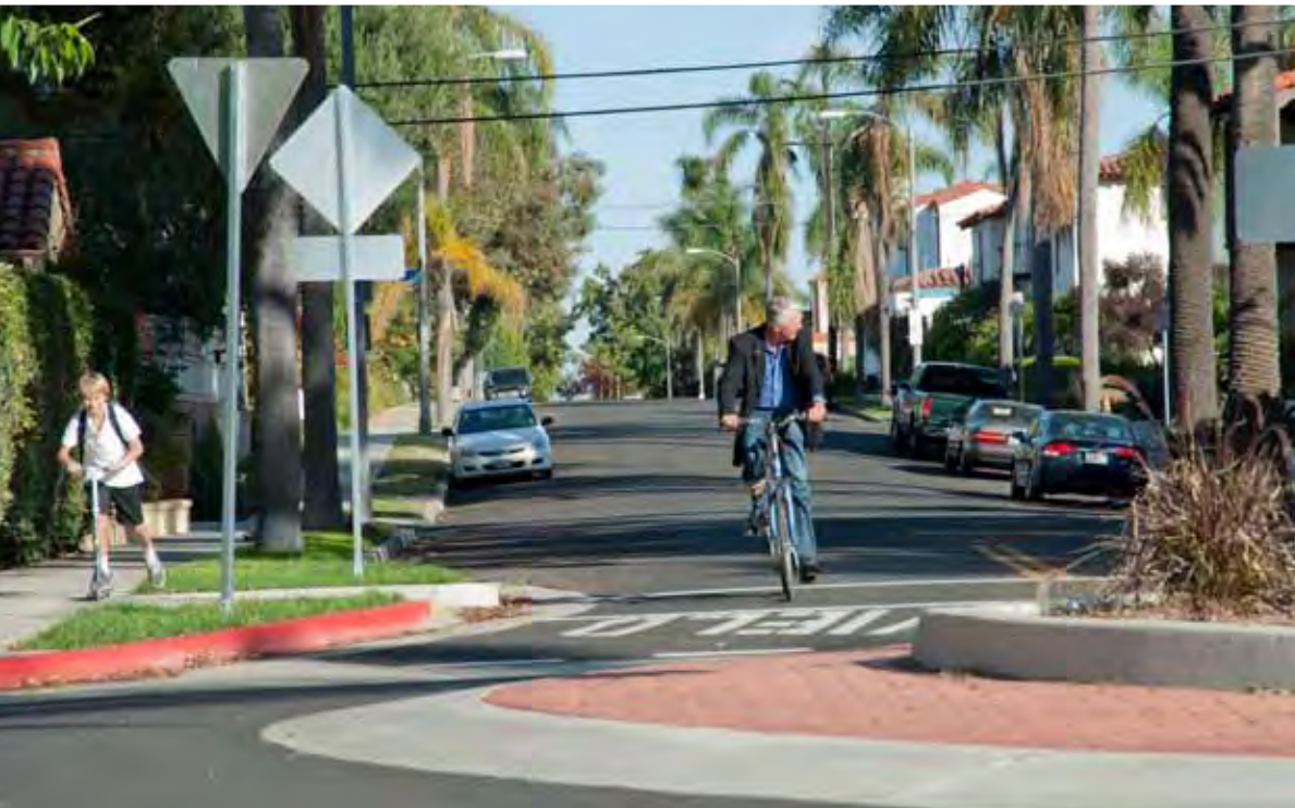
Roundabouts reduce vehicle speeds on residential streets and provide convenient movement for bicyclists.
