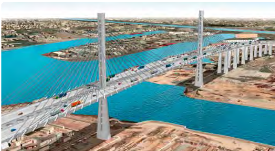
Gerald Desmond Bridge replacement.
