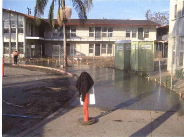
24 Affordable Units – Under Construction
