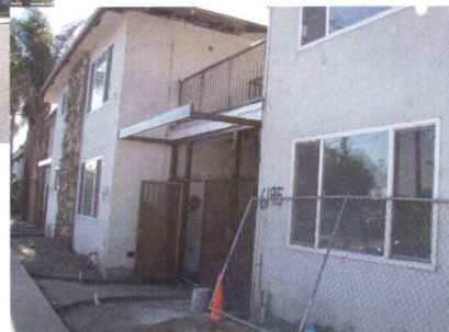
18 Affordable Units – Under Construction
