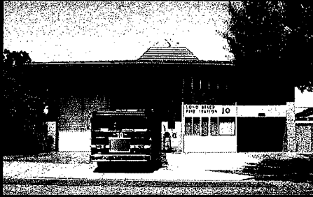
Fire Station 10 1417 Peterson Avenue Built in 1967
