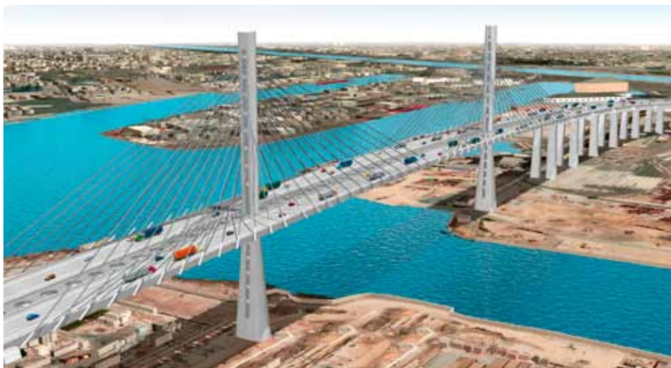
Gerald Desmond Bridge replacement.
