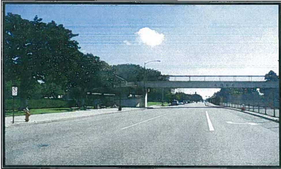
CORNER OF FACULTY & CARSON VIEW TOWARDS WEST (3)
