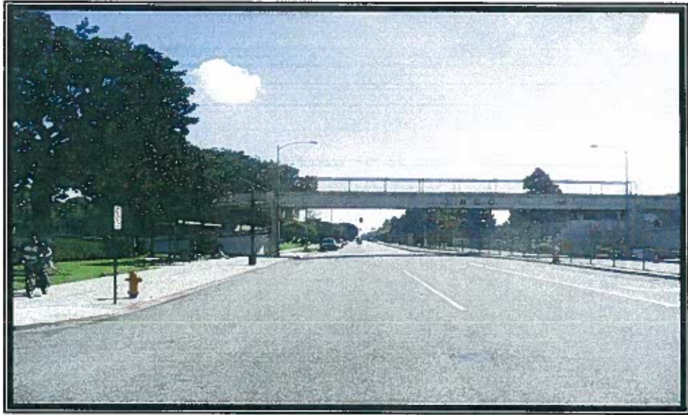
CORNER OF FACULTY & CARSON VIEW TOWARDS WEST (2)
