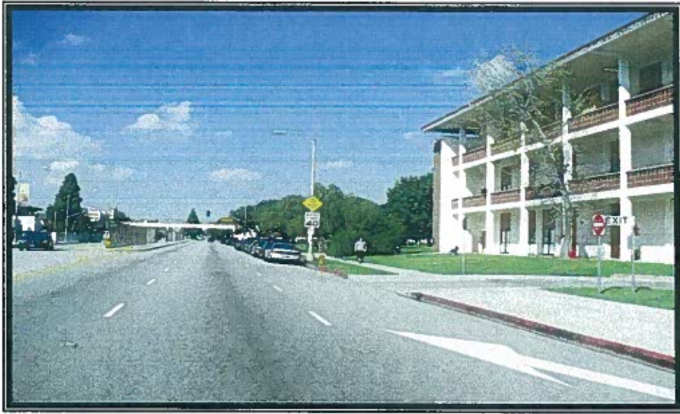
VIEW TOWARDS WEST ON CARSON (6)
