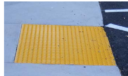
A set of yellow truncated domes can be seen on the down-ramp in a parking lot.
