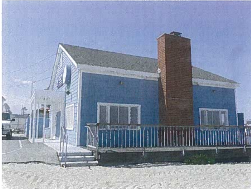
Figure 6: South elevation, looking north. Source: GPA.
