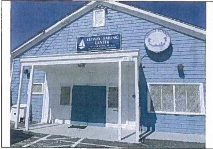
Figure 4: West elevation, looking east. Source: GPA.
