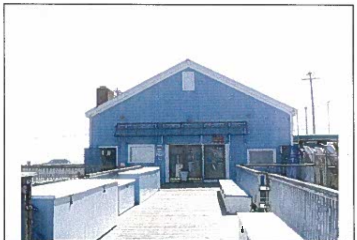
Figure 7: East elevation, looking west. Source: GPA.
