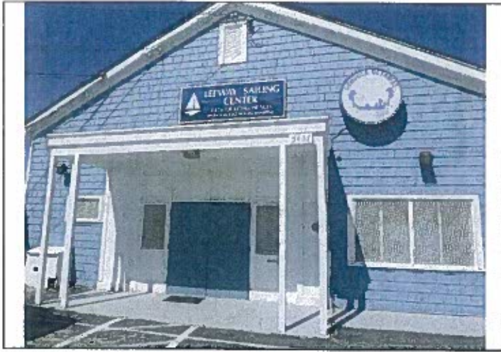
Figure 4: West elevation, looking east. Source: GPA.
