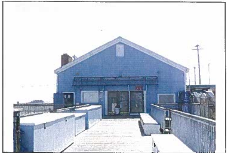
Figure 7: East elevation, looking west. Source: GPA.
