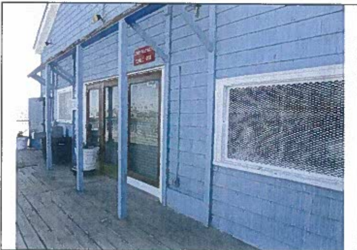
Figure 8: Detail view of east elevation, looking southwest. Source: GPA.
