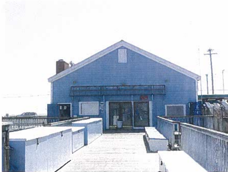
Figure 7: East elevation, looking west. Source: GPA.
