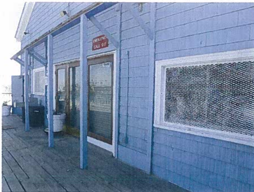
Figure 8: Detail view of east elevation, looking southwest. Source: GPA.
