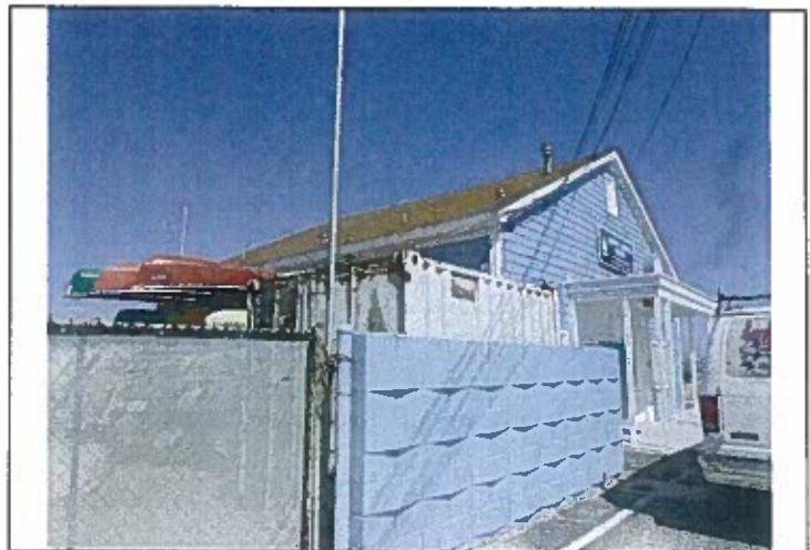
Figure 9: North elevation, looking south, view obscured by fence and storage. Source: GPA.
