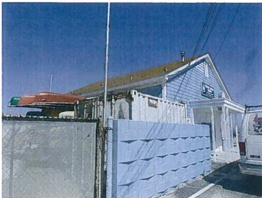
Figure 9: North elevation, looking south, view obscured by fence and storage. Source: GPA.
