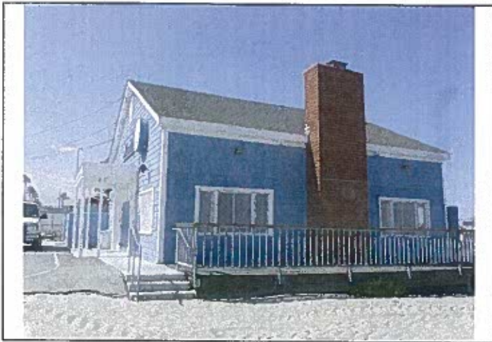
Figure 6: South elevation, looking north. Source: GPA.
