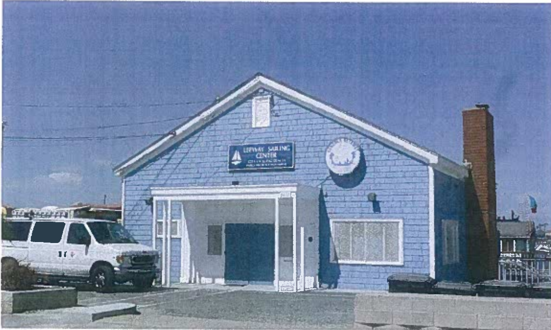
Figure 3: 5437 E. Ocean Boulevard, west elevation, looking east, April 2013; Source: GPA Consulting.
