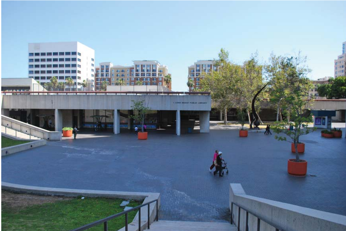
Photo 10: Looking South from Centennial Plaza at the existing Long Beach Public Library on the proposed project site.
