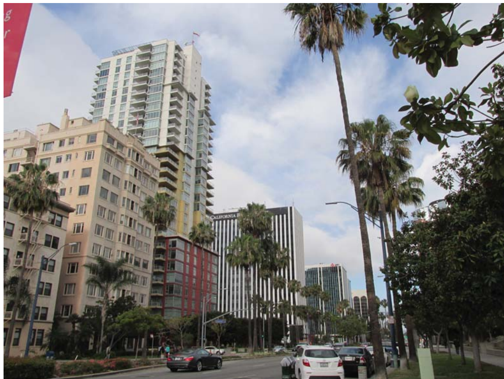
Photo 6: Looking West along Ocean Boulevard at surrounding residential and commercial buildings across from the project site.
