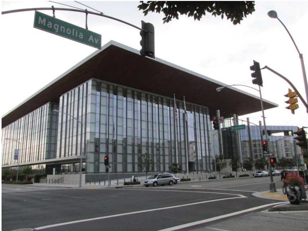
Photo 3: Looking Northwest from Magnolia Avenue and Broadway towards the Governor George Deukmejian Courthouse.
