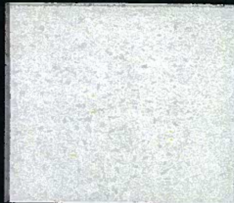
TOWER CORES / MAINTENANCE FACILITY ARCHITECTURAL CONCRETE
