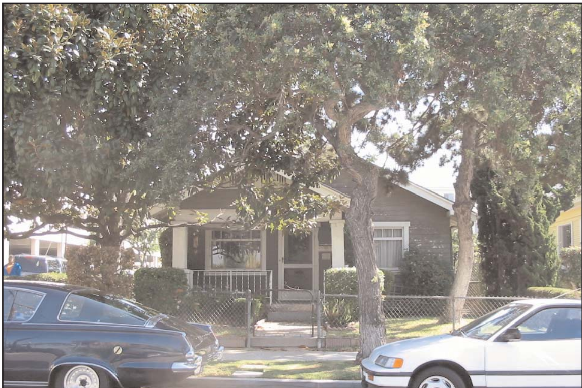
PHOTO 2 Photograph of 2690 Elm Avenue
