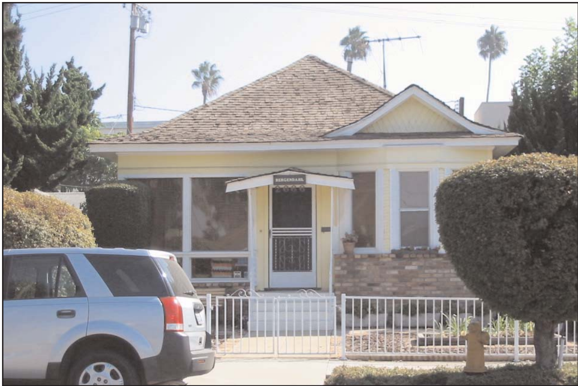
PHOTO 1 Photograph of 2666 Elm Avenue
