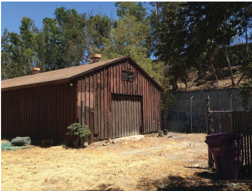
Photo 4: Abandoned storage building in southern part of project site, looking southeast, with UP Railroad berm and tracks in background
