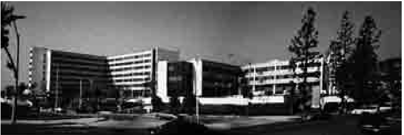
FIGURE 1.01 - Long Beach Memorial Medical Center and Miller Children's Hospital
