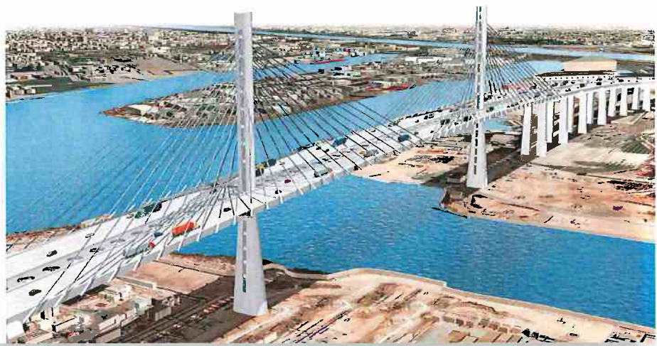
Gerald Desmond Bridge replacement.
