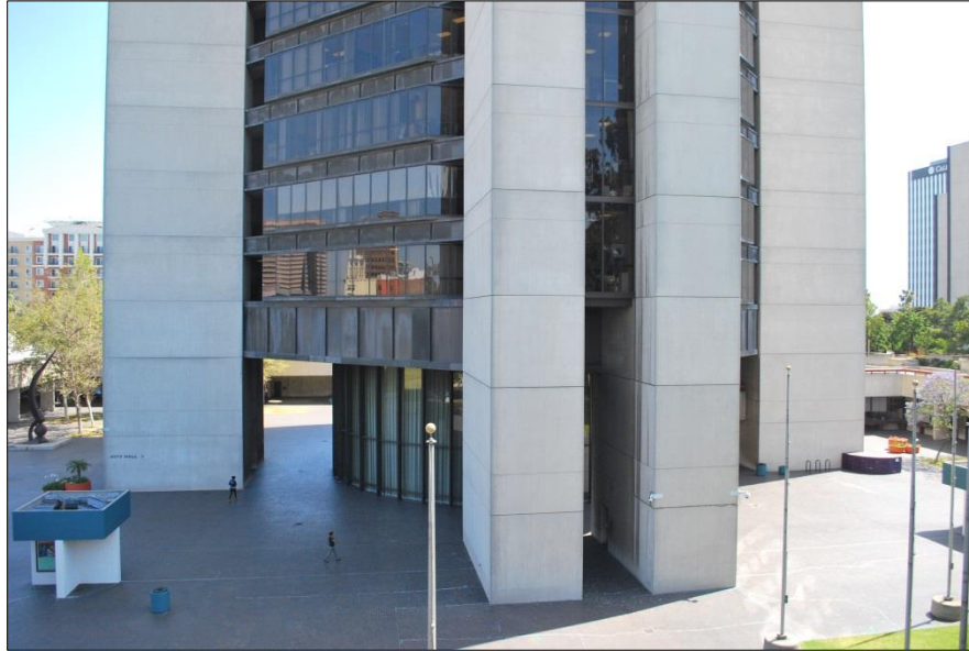
Photograph 2. City Hall, facing south.
