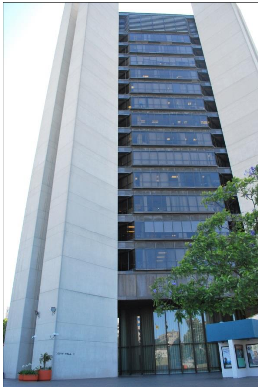
Photograph 1. City Hall, facing south.
