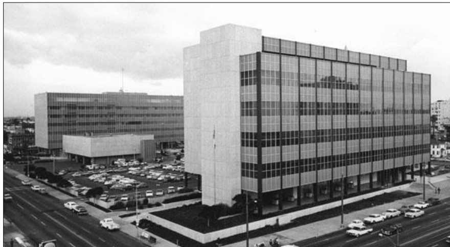
Figure 10. View northeast of Courthouse and Public Safety Building, 1960. Source: City of Long Beach Library
