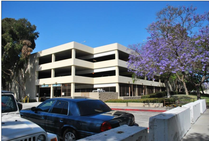
Photograph 15. View northeast of Parking Garage.
