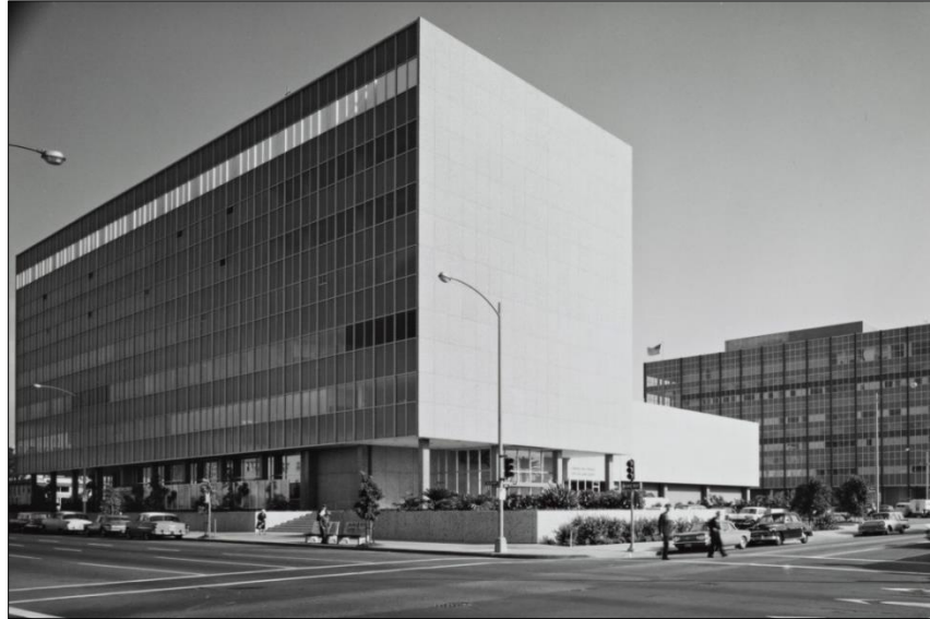
Figure 8. View southeast of Public Safety Building, north and west elevations, 1961.
