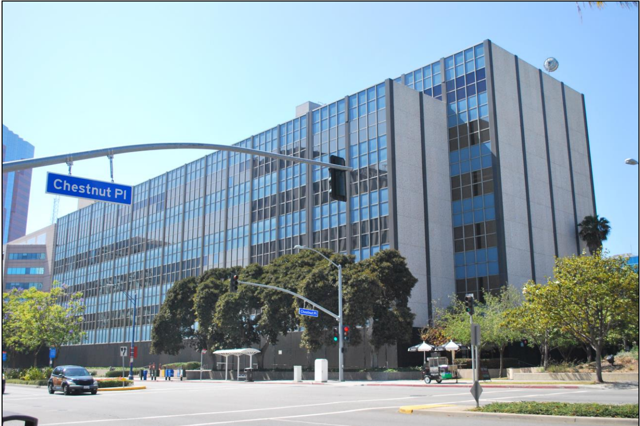
Courthouse, view to the northwest. 5/12/2015
