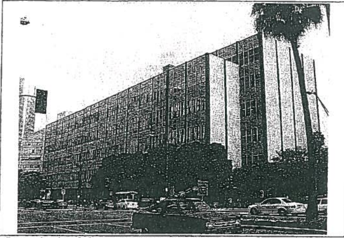
Image 1: View facing northwest at south-facing façade
