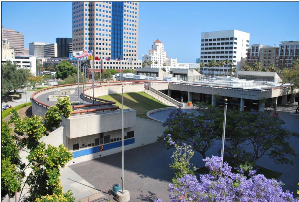
Photograph 5. Library facade, facing southeast.
