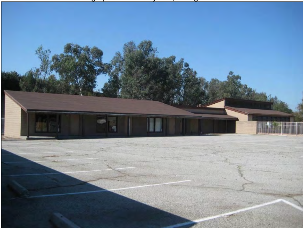
Photograph 4. Training Center, facing south
