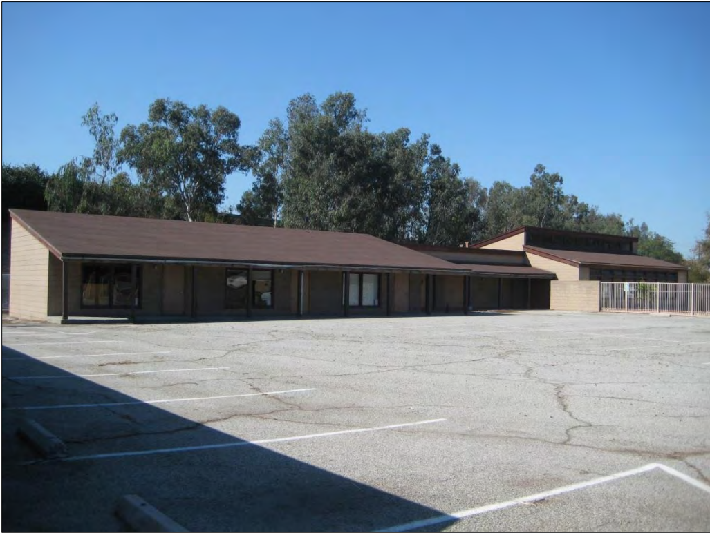
Photograph 4. Training Center, facing south.
