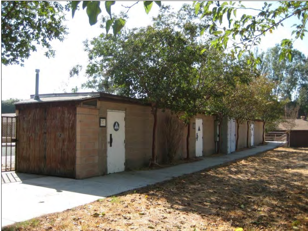
Photograph 7. Changing Rooms, facing southeast.
