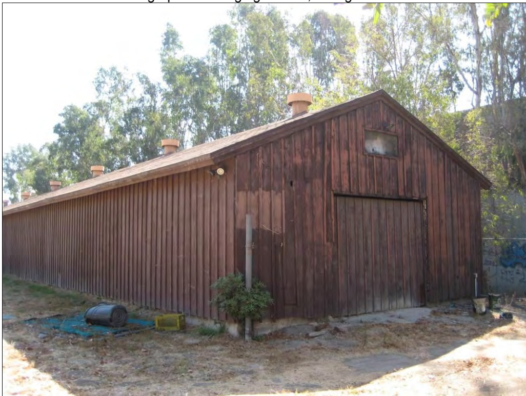
Photograph 8. Storage Building, facing southeast.
