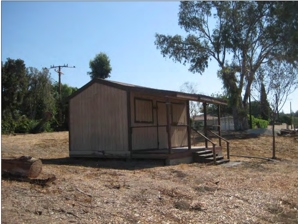
Photograph 9. Camp Master building, facing northeast.
