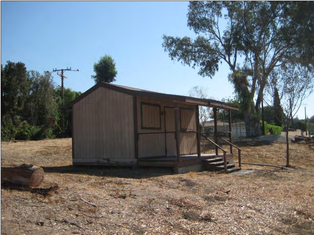
Photograph 9. Camp Master building, facing northeast.
