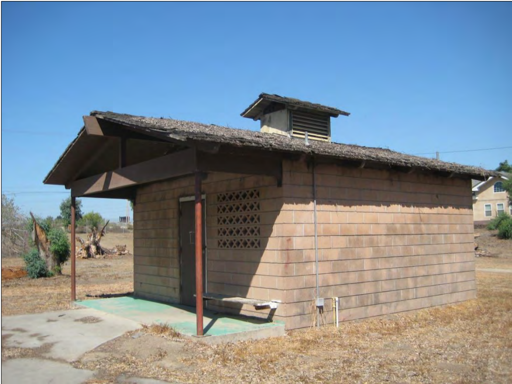
Photograph 12. Restroom, facing northwest.
