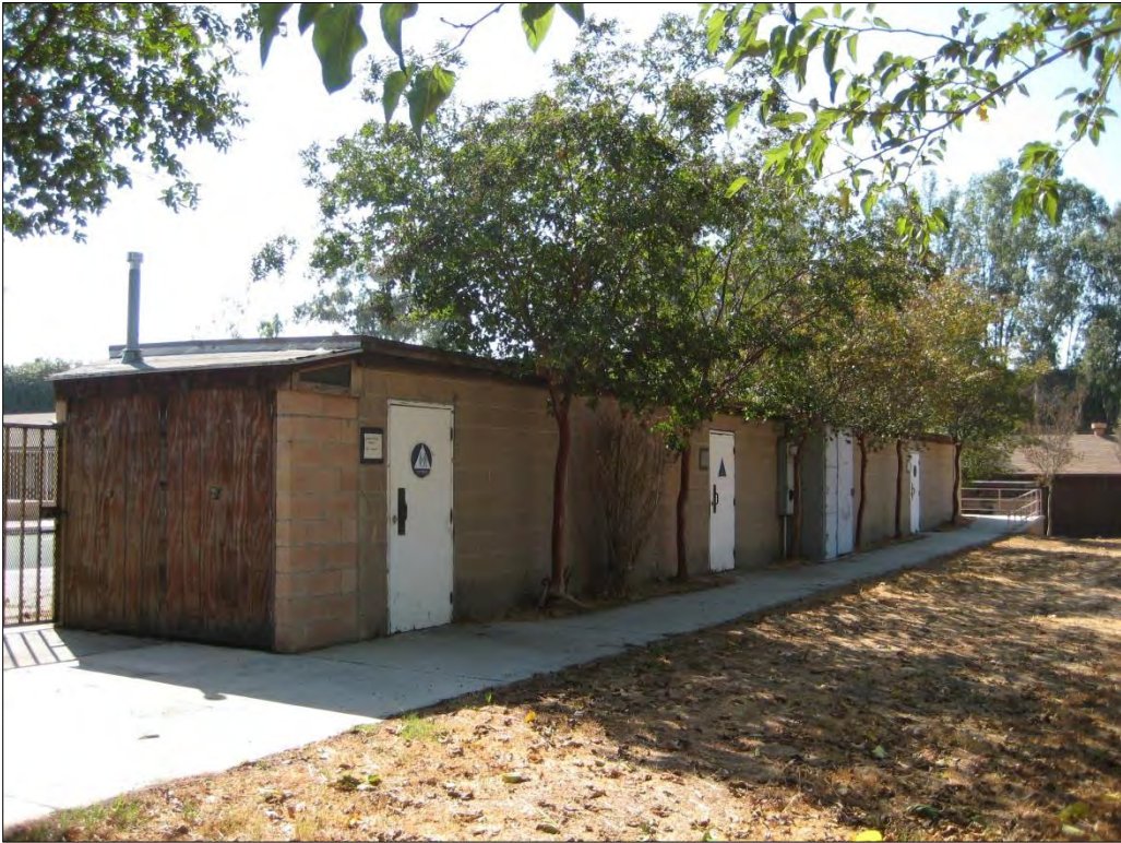
Photograph 7. Changing Rooms, facing southeast.
