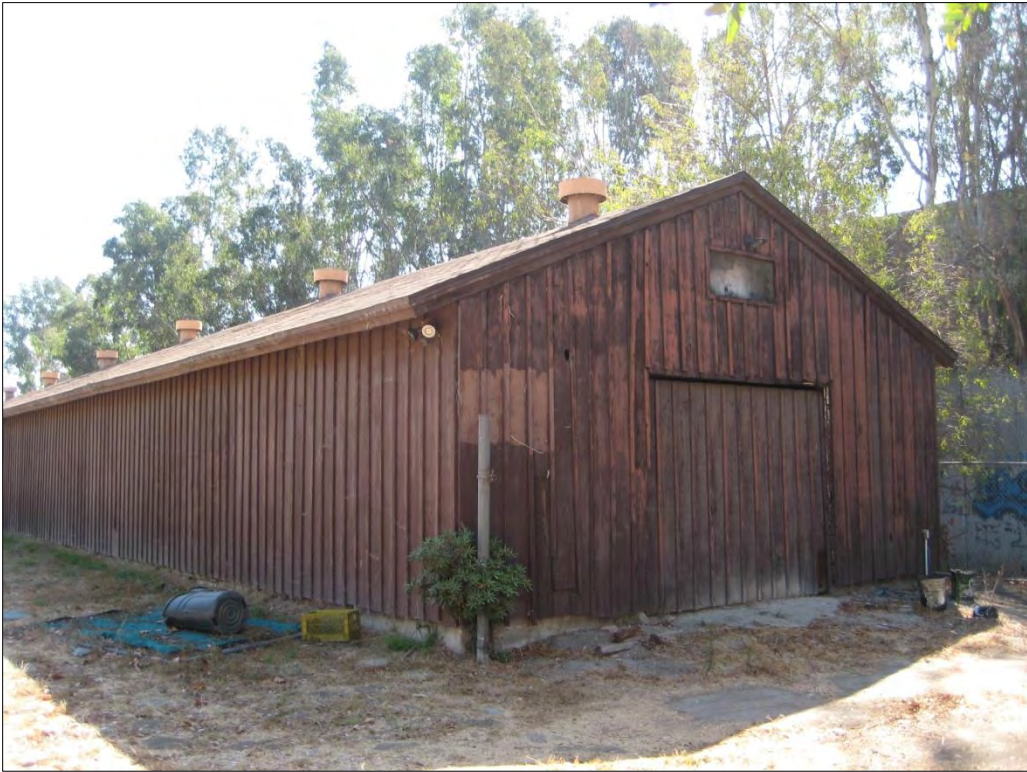
Photograph 8. Storage Building, facing southeast.
