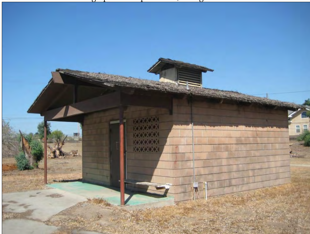
Photograph 12. Restroom, facing northwest.
