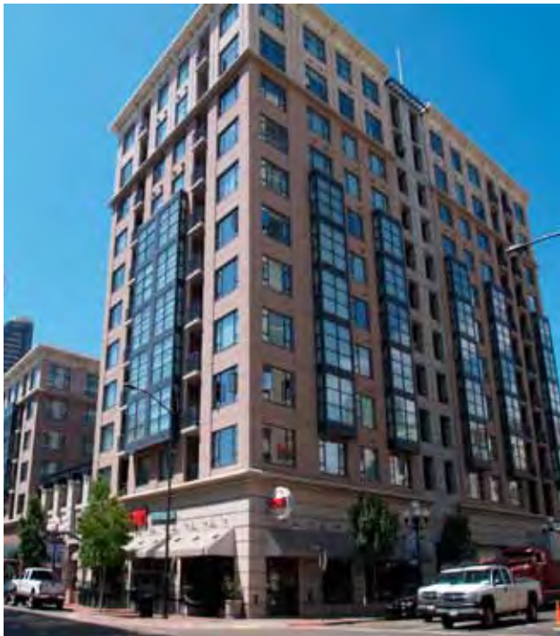
Example of high-quality materials used on a new mid-rise building that exhibits a classic base, middle and top composed of more substantial material and storefront details at the pedestrian level, plus inset balconies and a variety of window types.
