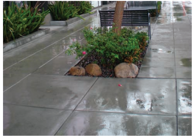
Pavers may be used within the right-of-way if they are earth-toned and have only subtle variations in color. Pavers shall be square or rectangular and a minimum size of 8 inches by 8 inches.
