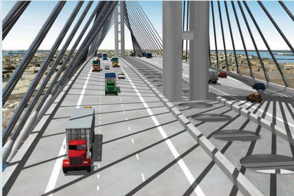
The proposed Gerald Desmond Bridge replacement would have three traffic lanes in each direction, plus dedicated emergency lanes to reduce traffic delays and safety hazards from accidents and truck breakdowns.
