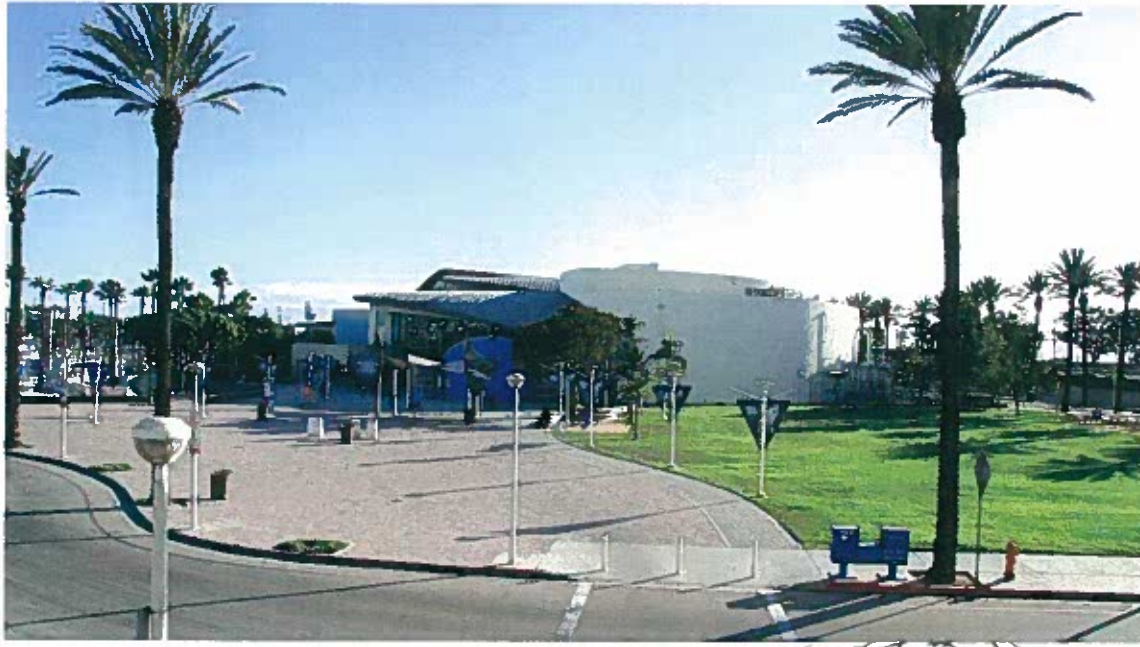
Perspective of existing entrance from parking structure
