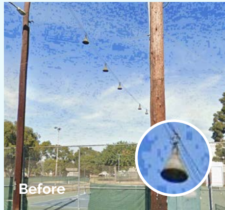
Left: team installs wiring for new L.E.D. tennis court lights. Center: Old 1930's festoon type lighting. Right: six new LED poles and fixtures light up the courts at Silverado Park.
